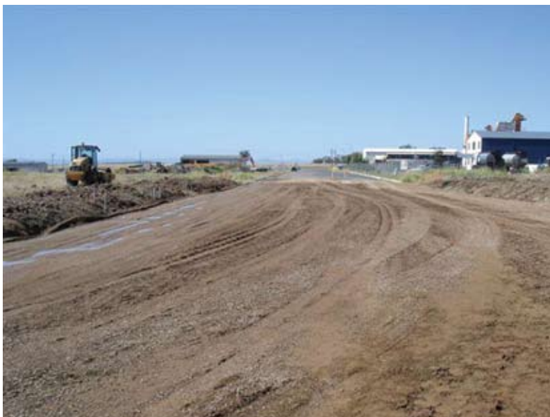
Photo 5. Recycled Sub-base ready for compaction
