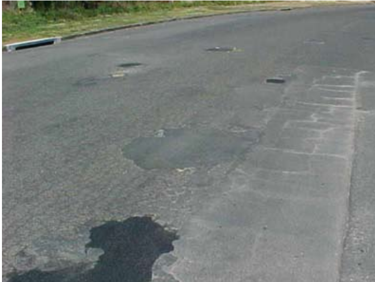
Photo 2. Delgarno Road before reconstruction
