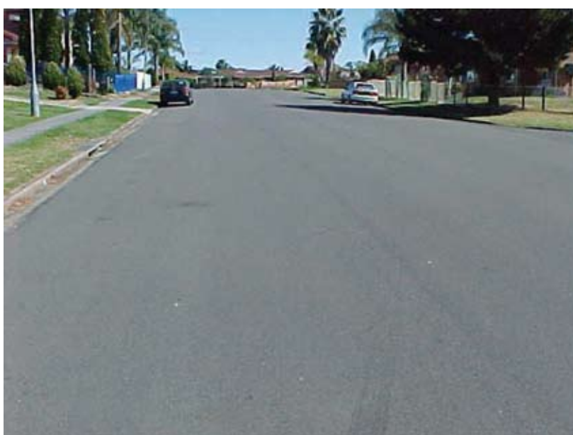
Photo 3. Delgarno Road – Road condition 7 years after the rehabilitation work
