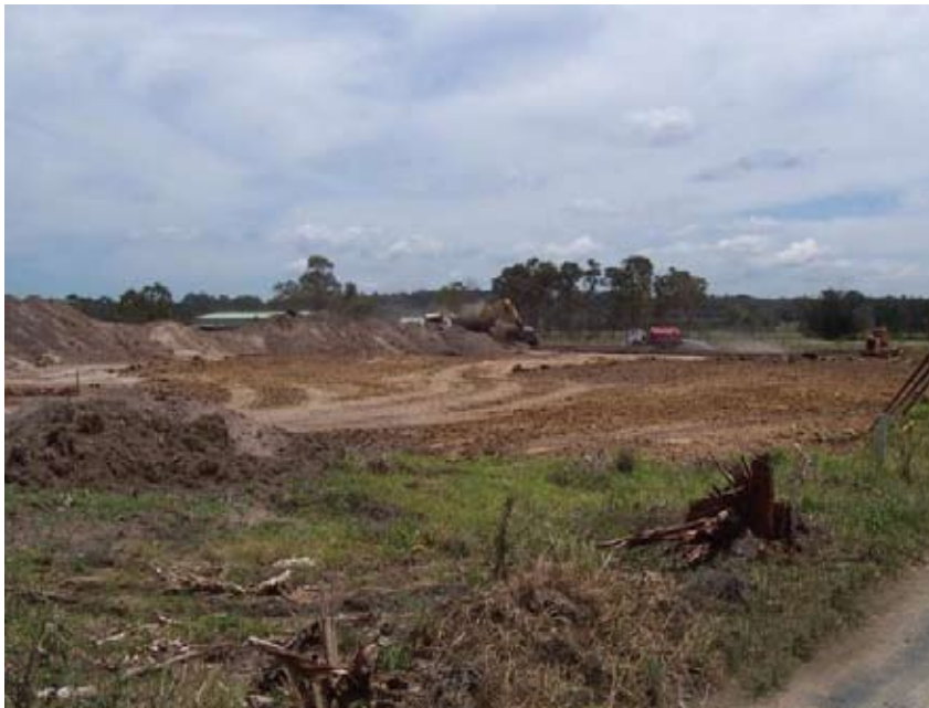
Photo 7. Early site works
