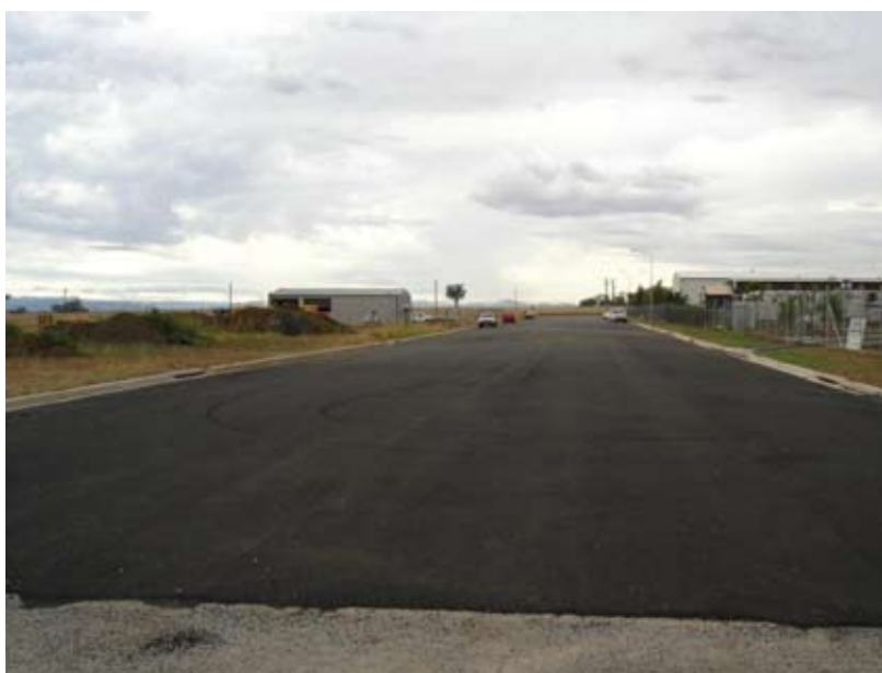
Photo 6. Completed, sealed Armstrong Street
