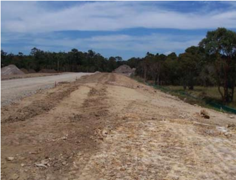
Photo 8. Site Filling and Recycled Concrete – Note depth of Fill
